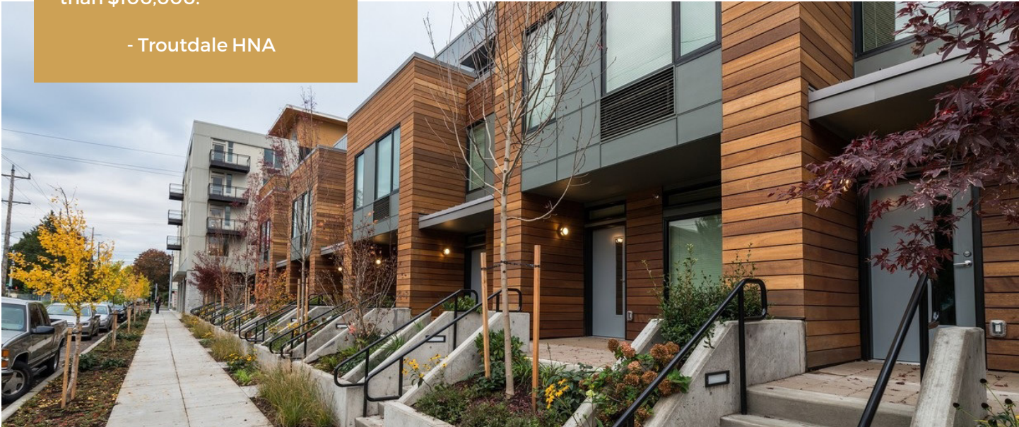
Peloton Apartments and Townhomes, Portland, OR
