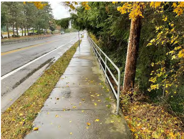
Image 9: Arata Creek Crossing Under NE Halsey Street Near Donald L Robertson City Park
