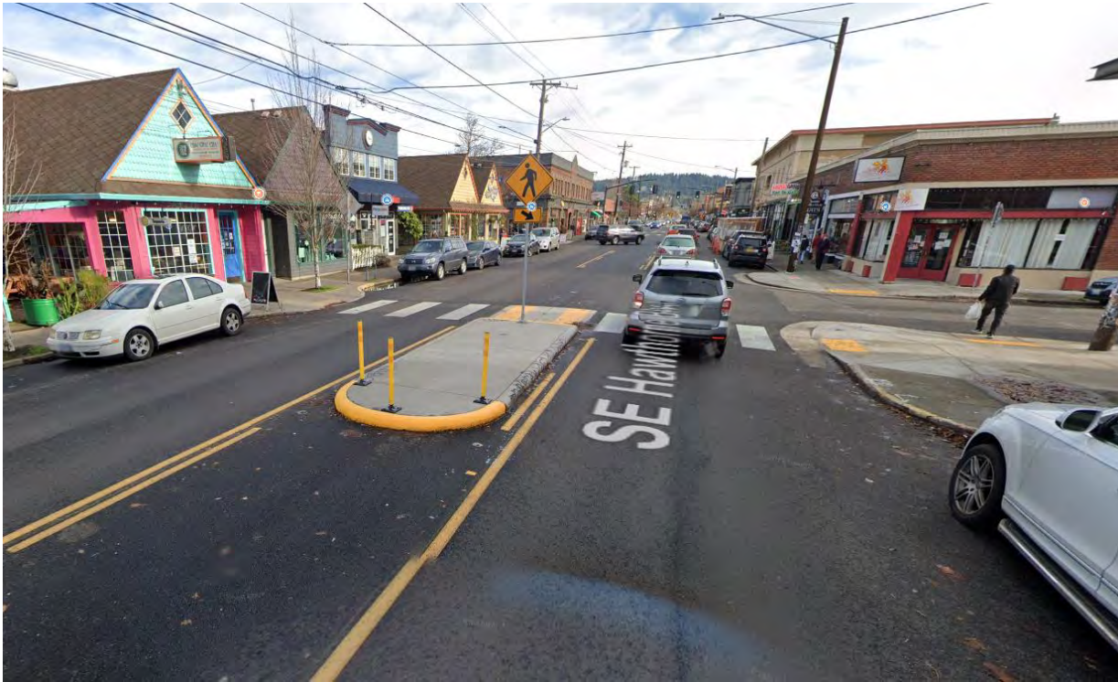
Figure 21. Example Pedestrian Crossing with a Refuge Island and Curb Extensions (Portland, Oregon)
