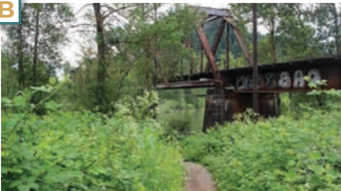
Current access to the site under the railroad trestle to the site, connecting to the future bike hub, visitor's center and Downtown
